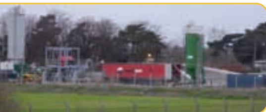
Anglia Water's Flag Fen water treatment plant in Peterborough: using a mobile decanter to supplement treatment facilities on plant
